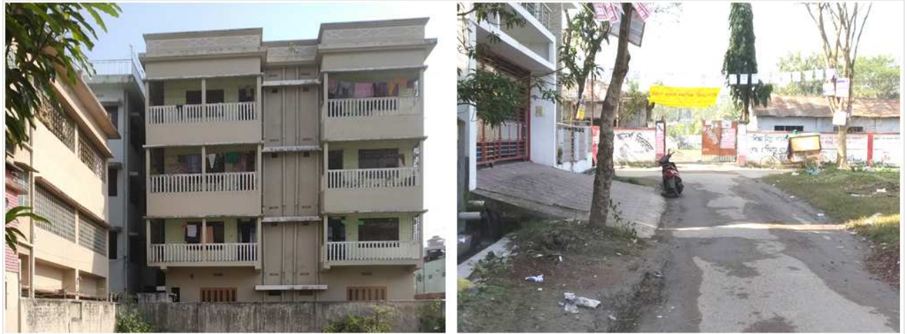
Fig. 2a. Violation of setback regulation, Fig. 2b. Car parking ramp connected to the road
