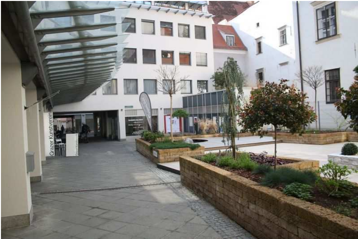
Fig 5.: The inner courtyard in the Bürgergasse 5. building
