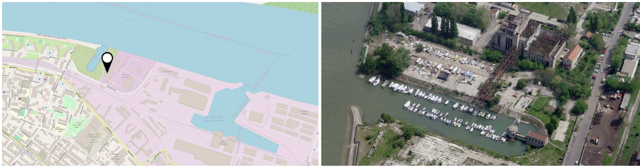
Fig. 3: The position of the Thermal Power Station in relation to the immediate environment (left) and the aerial view (right).
