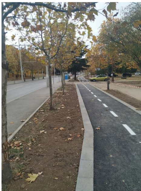
Fig.3 The new sidewalk along “V. Levski” Boulevard
