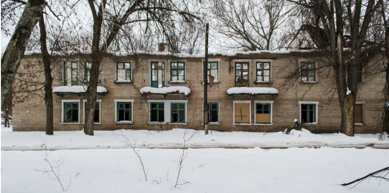
Fig. 2: A dilapidated apartment building, whose residents were relocated according to the housing program. Photo: M. Bolotov, 2020
