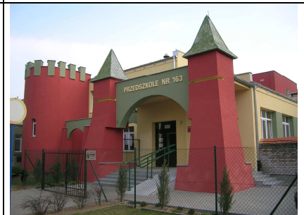
Figure 18. Renovation of a public infrastructure – a kindergarten
