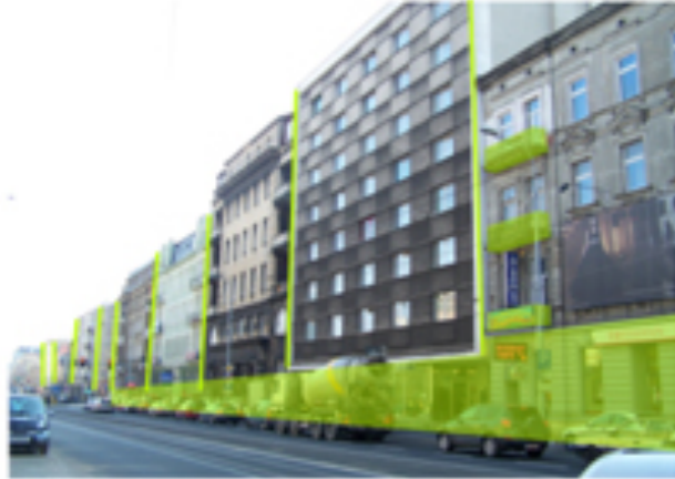
NORTH FRONTAGE OF NARUTOWICZA STREET
