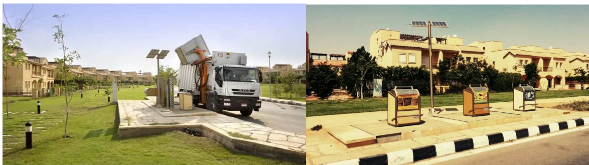
waste management and solar panels
